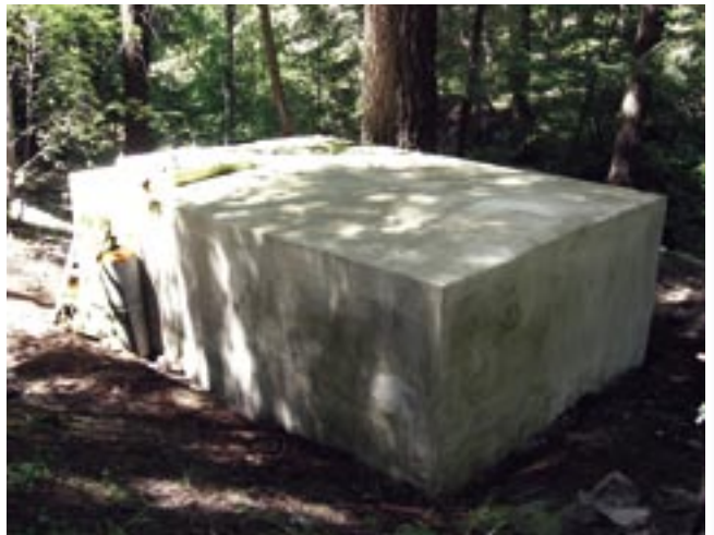
Figure 33—Concrete water tank.
