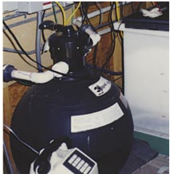
Figure 78—Manually backwashed rapid sand filter.
