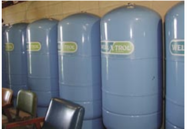
Figure 31—Pressure tanks.
