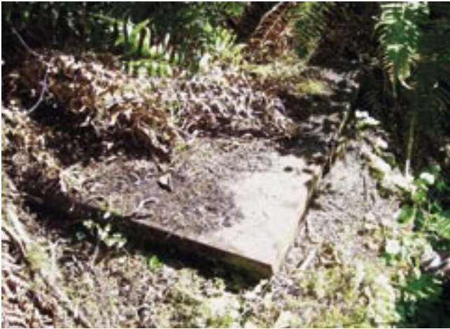
Figure 20—Clear brush and grade to drain.
