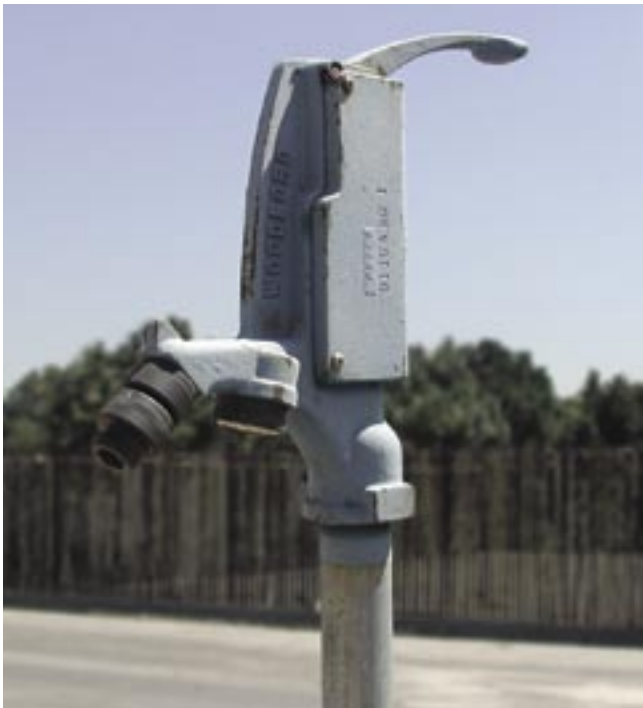
Figure 44—Freezeproof hydrant.
