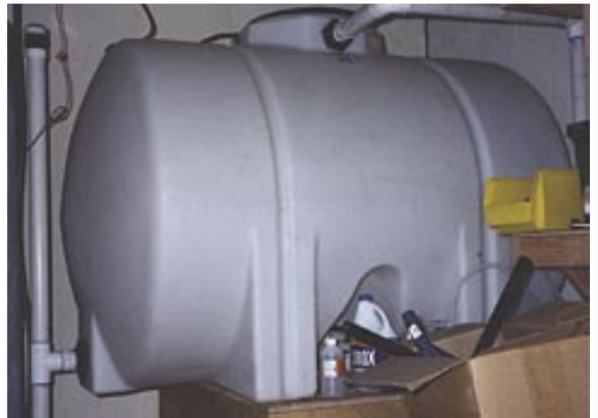
Figure 32—Polyethylene tank.
