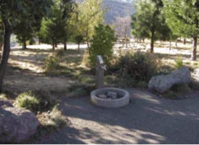
Figure 47—This armored splash zone allows drainage and prevents site erosion.
