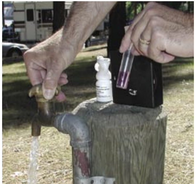
Figure 54—Test water for free chlorine.
