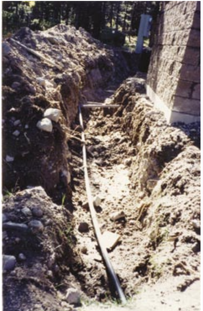
Figure 39—Distribution system pipe placed in a trench.
