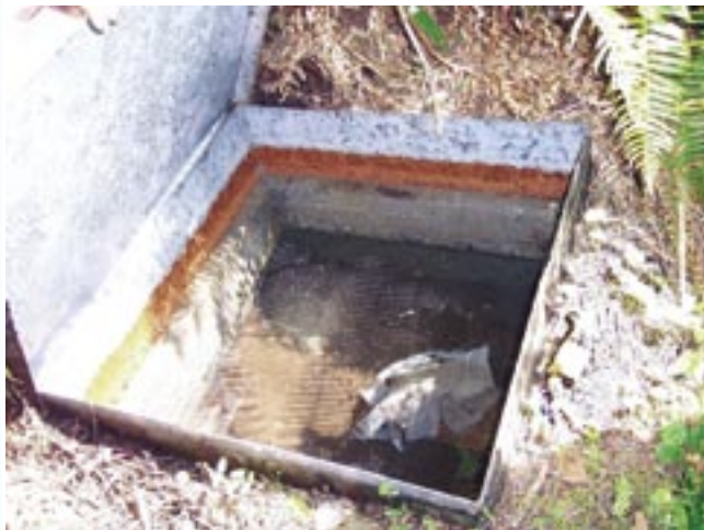
Figure 29—Clean debris from the spring box and repair the lid seal.
