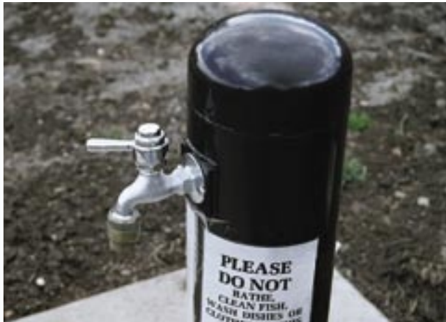
Figure 84—Atmospheric vacuum breaker.
