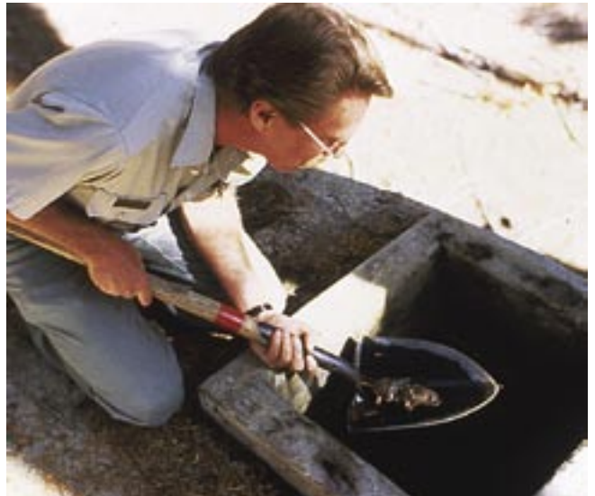
Figure 86—Tank contaminated by a dead rodent.
