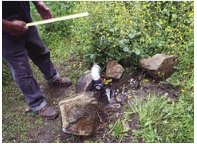
Figure 57—Drain all water lines.
