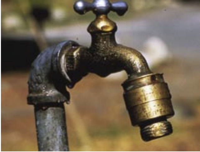
Figure 43—Hose bib with vacuum breaker.
