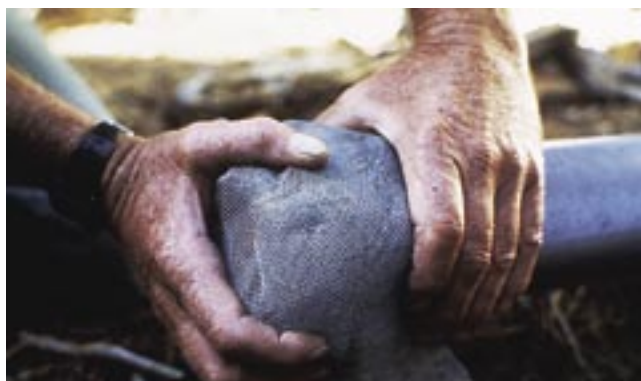
Figure 25—Replacing screen.
