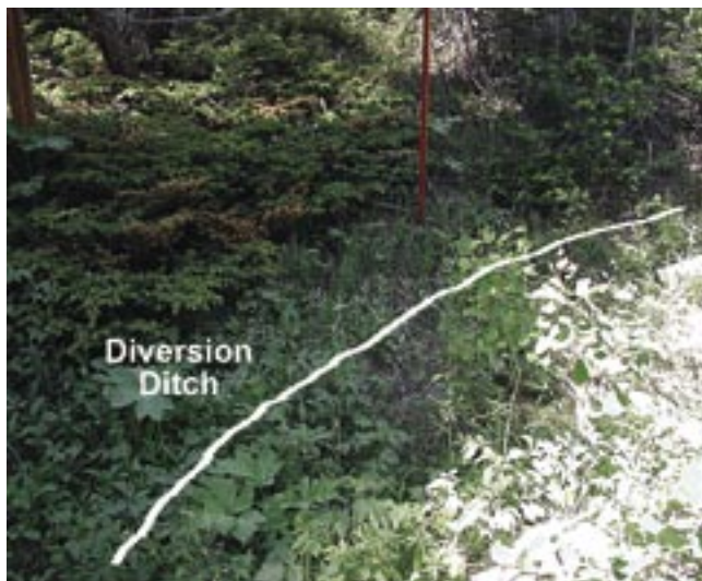
Figure 27—Diversion ditch.
