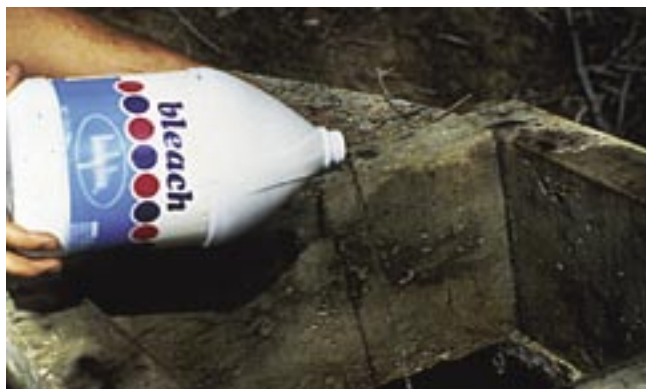
Figure 52—Shock-chlorinate seasonal systems. (Non-NSF bleach can be used for shocking the system as long as it is not scented and the water is not for human consumption.)
