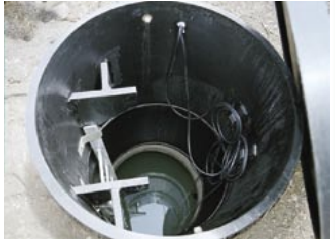
Figure 50—Open tanks and check for damage.
