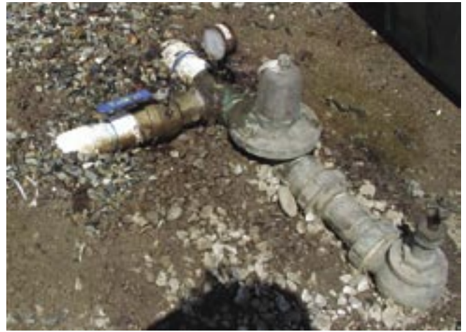
Figure 42—Leaking valve.
