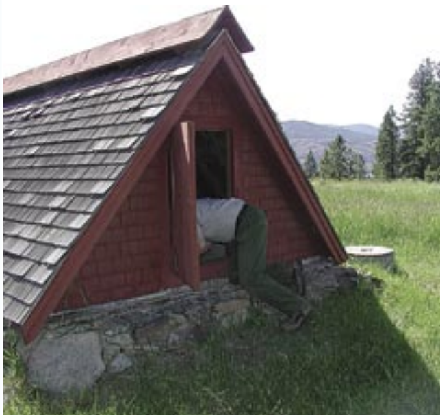
Figure 28—Check for damage to the spring's water collection and storage system.
