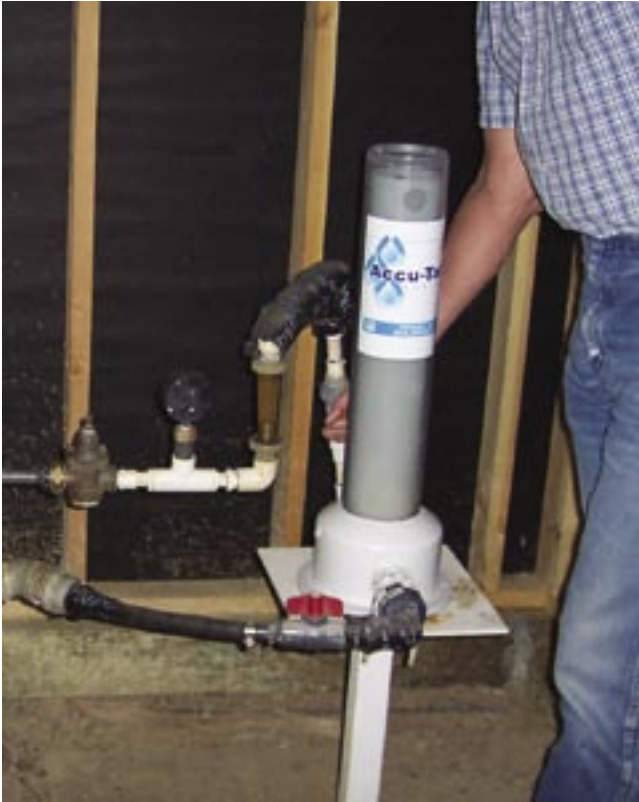
Figure 61—Erosion-feed chlorinator.
