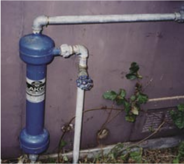
Figure 72—Centrifugal type filters remove heavy particles, such as sand, by spinning the water to create a vortex.
