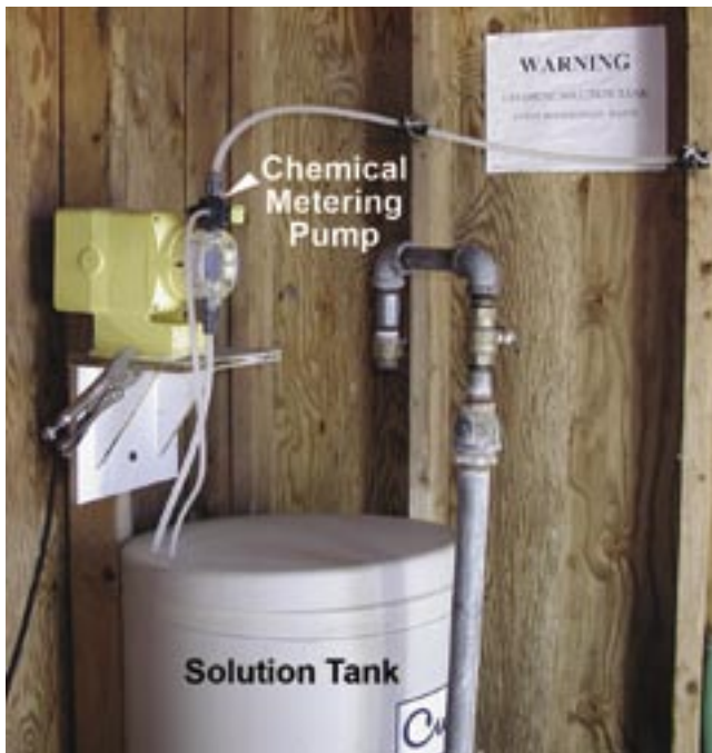
Figure 69—Hypochlorination system.
