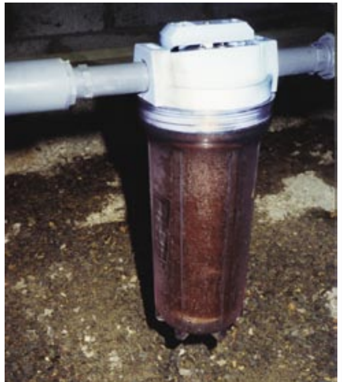
Figure 74—Small cartridge filter.
