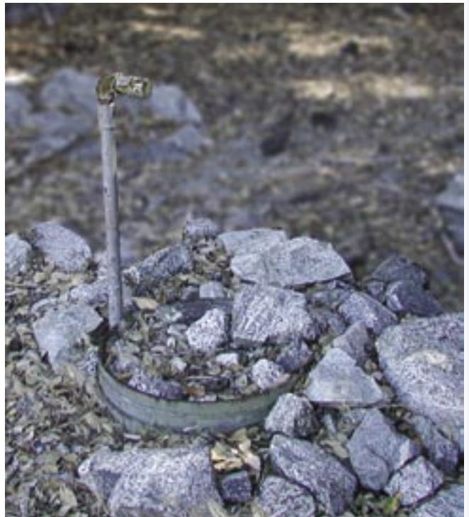
Figure 58—Cap lines when components are removed to keep pipes clean.
