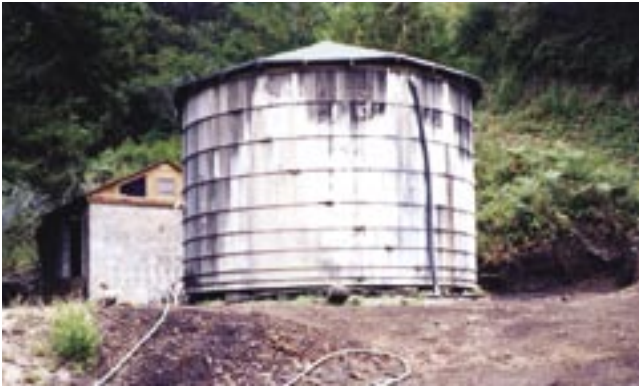
Figure 34—Wooden water storage tank.
