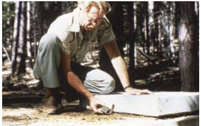
Figure 23—Spring box lid must be locked.
